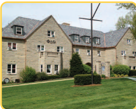
Gutters are being installed as we look forward to the finished roof.
